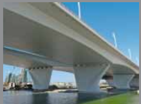
Al Garhoud Bridge, Dubai (AE)
